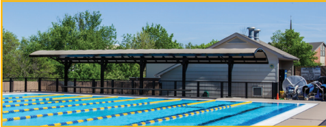
The Rockwood Swim Club 50-meter outdoor pool at Crestview Middle School was recently renovated and is our training facility from April through October.
